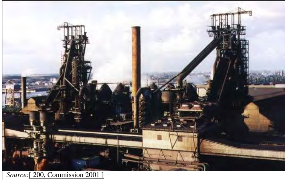
Figure 6.1: General view of two blast furnaces with three hot stoves each and the stack for the waste gas from the hot stoves
