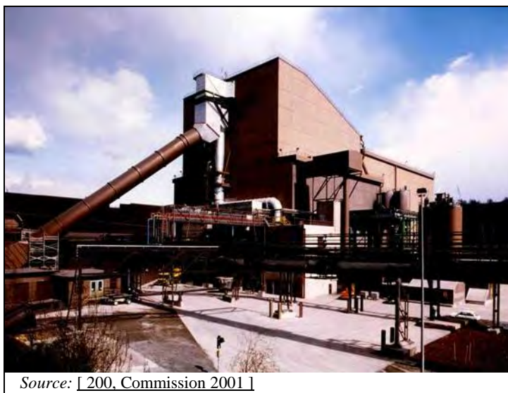
Figure 8.1: Electric arc furnace plant
