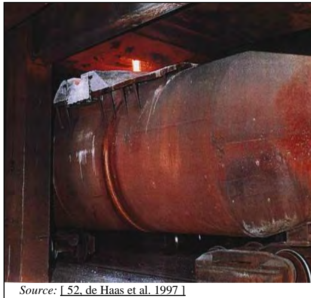
Figure 6.16: Charging of hot metal into torpedo ladle with dust suppression with inert gas
